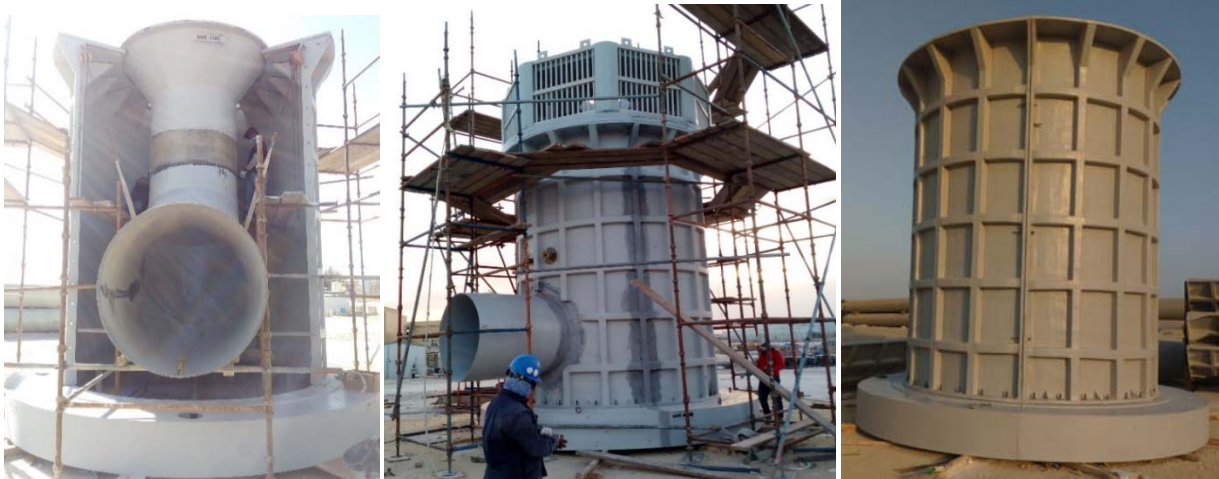
Figure 5: Vertical body with pipe before and after assembly of modular parts(KSA)
