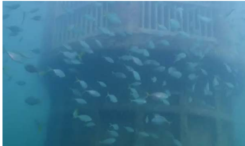
Figure 2: Fish swimming safely around GRP Intake tower (Kingdom of Saudi Arabia)
